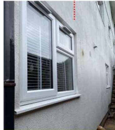
Figure 5 - New window positioned far south on the eastern elevation
