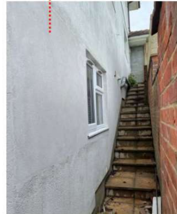
Figure 6 - New window positioned within former window opening
